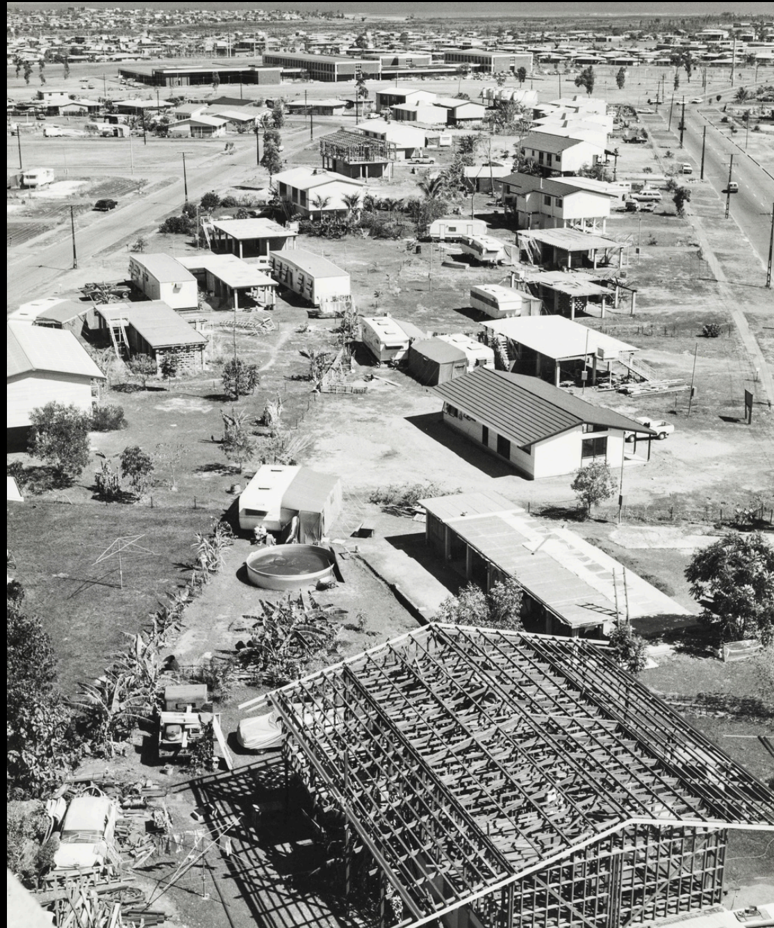
View from the Parer Drive water tower showing houses under construction or repair in Moil, January 1976.
